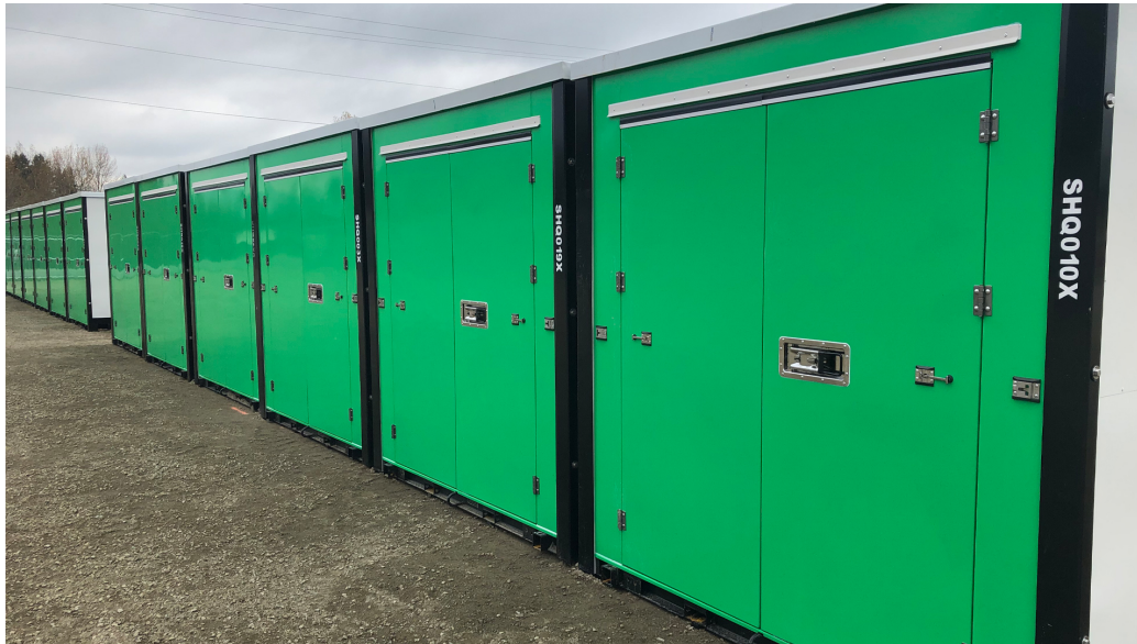
Existing Storage HQ storage units in Duncan, British Columbia
