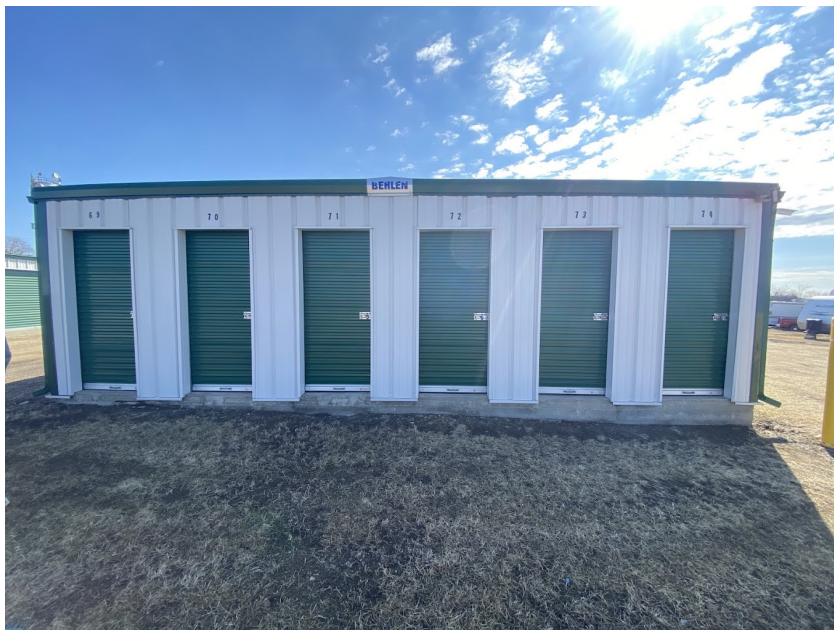
Existing Legal Self Storage units in Legal, AB T0G 1L0, Canada
